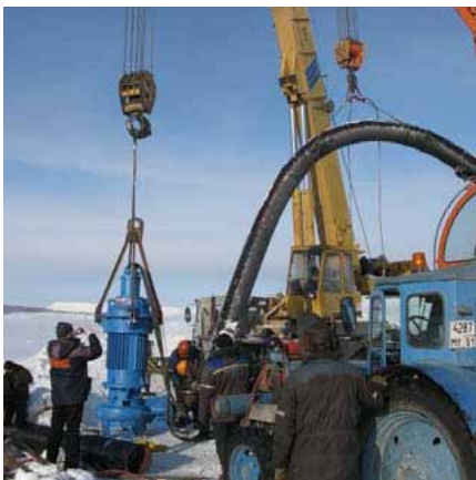
Warman® SHW pump installation, replacing a horizontal pump in a tailings dewatering application
